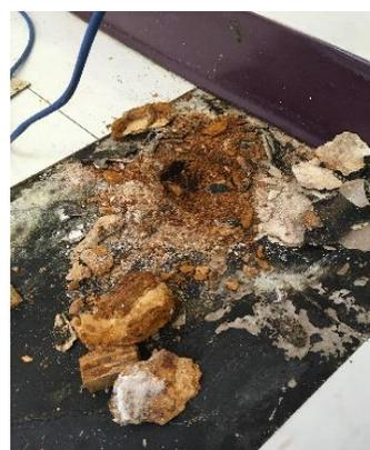
**Image 1.2** Water damage under lower-level tiles
