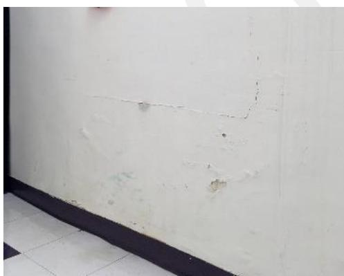
**Image 1.1** Lower level- Water damage on wall
